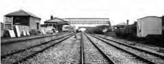
Ardley Station (now demolished) with the B430 bridge beyond. The cattle pens would have been on the left. Copyright: Packer/ Oxfordshire History Centre
