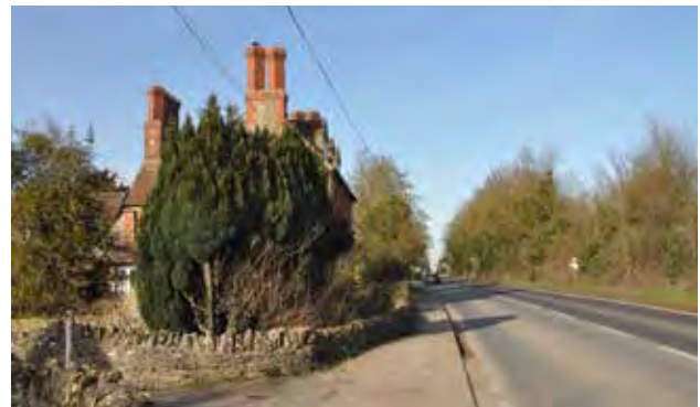
Looking north to Jersey Cottage on Station Road
