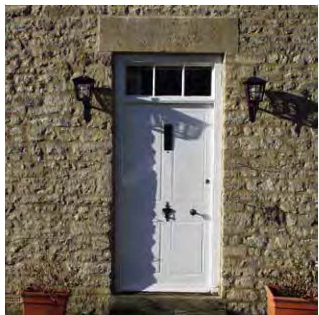
Painted timber panelled door with flush beaded panels and simple overhead
