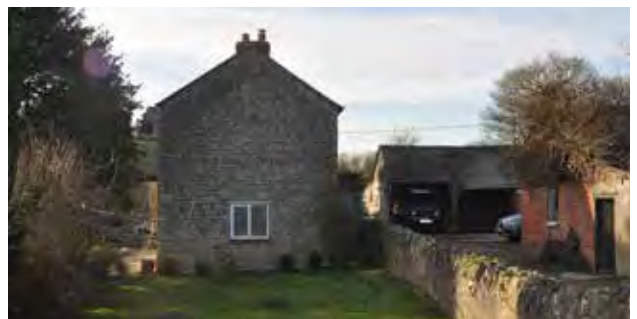
Woodview Cottage and outbuildings
