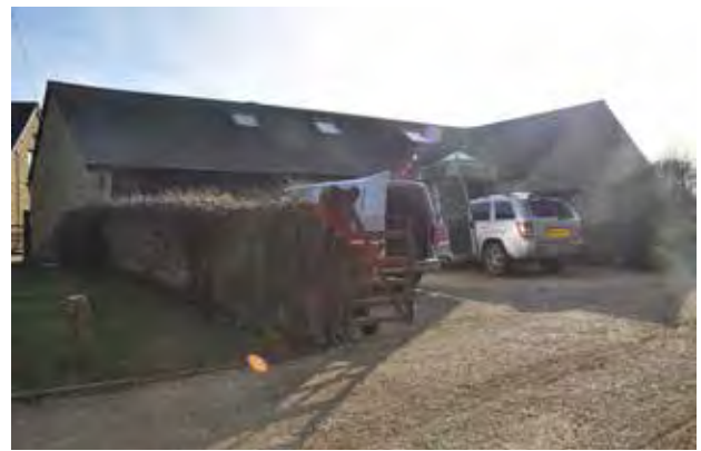
Manor Barn (former open shed for cattle)
