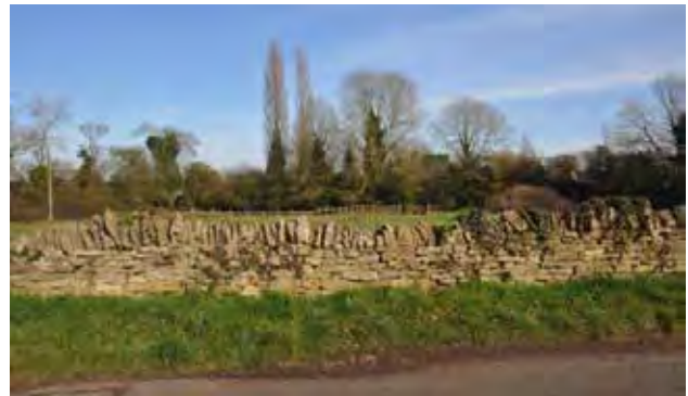
Stone wall to the field north of Ardley House
