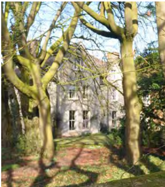
Painted timber sash and case windows at Ardley House
