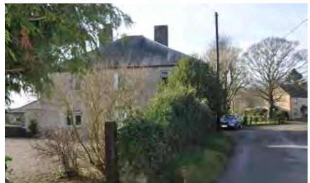
13. Church Cottage, Church Road
